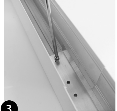
3 Tighten 4x screws.
