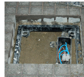
RAD 250 Buried uplight installation 1 Installation sleeve and wiring box are fitted at the first fix.
