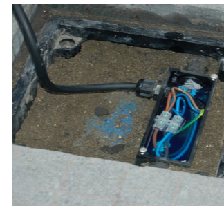
RAD 250 Buried uplight installation 3 Luminaire installation Luminaire cable connected and flexible gel added to wiring box to achieve a water proof seal. The gel remains soft and can be removed to allow the luminaire to be disconnected for servicing at any time after installation.
