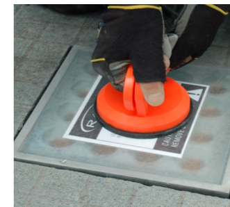
RAD 250 Buried uplight installation 3 Luminaire installation Luminaire cable connected and flexible gel added to wiring box to achieve a water proof seal. The gel remains soft and can be removed to allow the luminaire to be disconnected for servicing at any time after installation.
