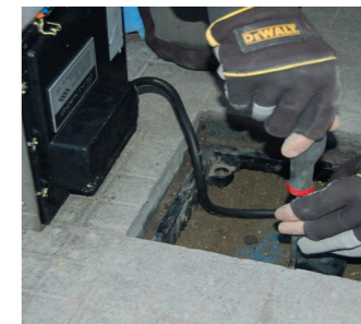
RAD 250 Buried uplight installation 1 Installation sleeve and wiring box are fitted at the first fix.
